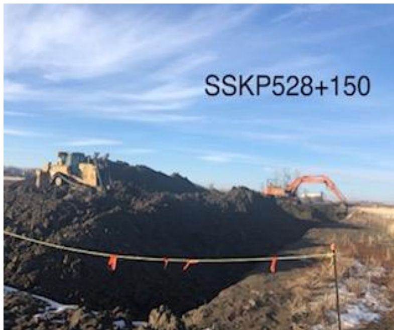
Backfill test site at Kick off
